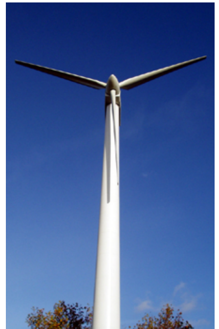
Renewable energy generation
